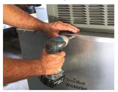
4. Lift out the insulation pad.
