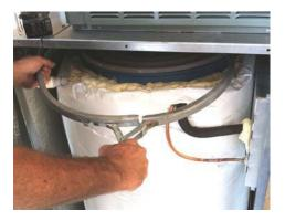
6. Lift off and remove the Chiller Barrel lid.
